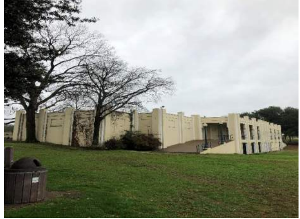
Bath House Cultural Center
