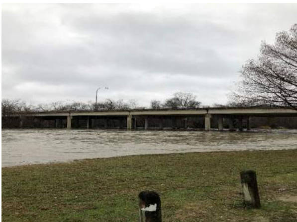
Mockingbird Road Bridge
