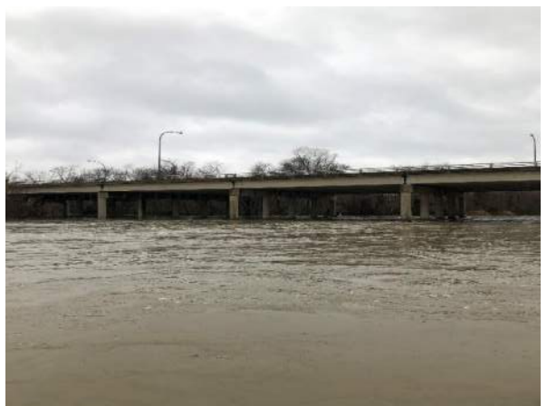
Mockingbird Road Bridge
